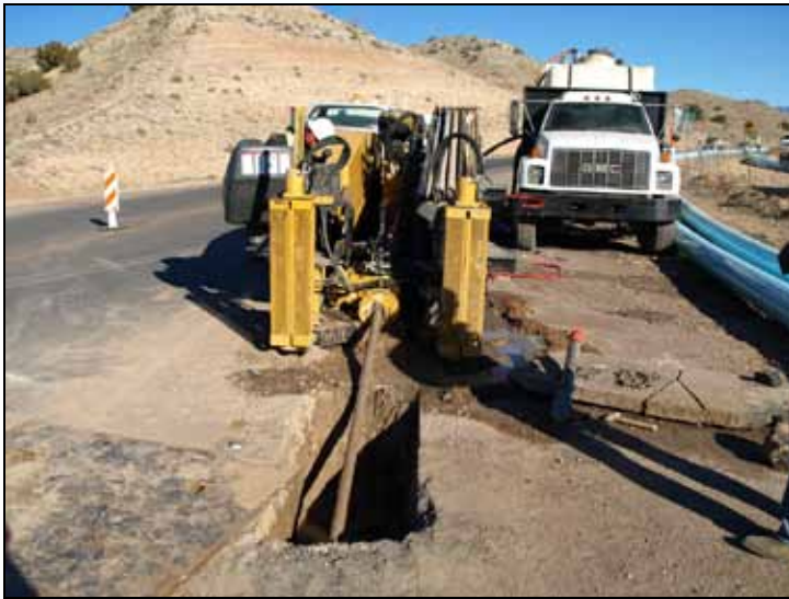
Directional drilling rig for HDD
